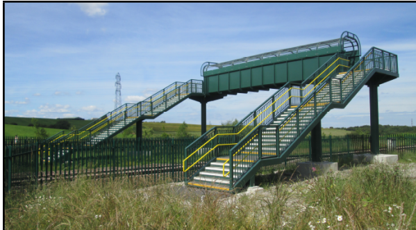
Figure 2: An example of a stepped structure
